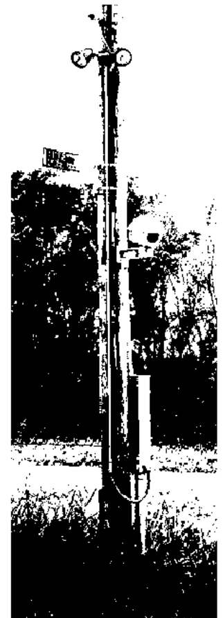
Various items on utility pole (Image source: unknown)
