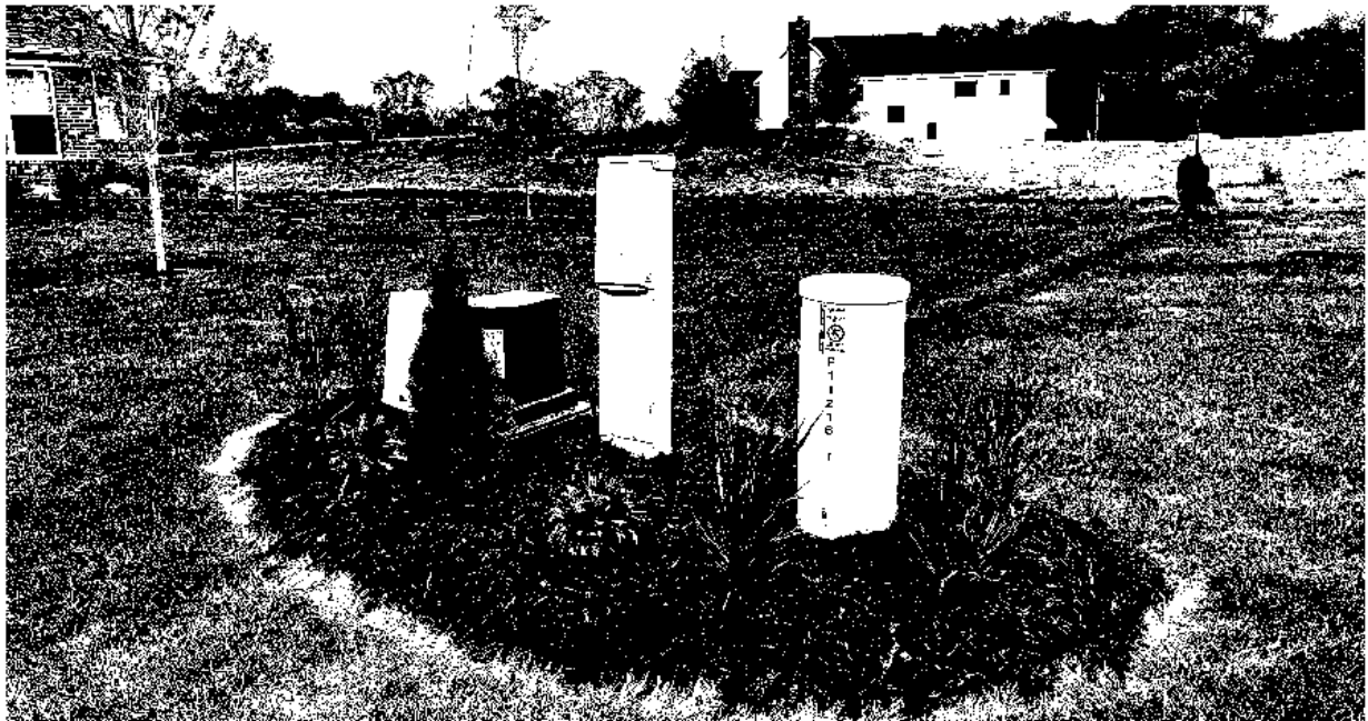
Typical underground utility “cluster” (Image source: unknown)
